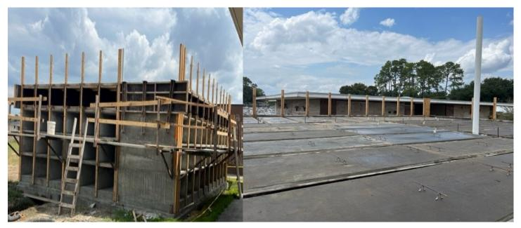
The construction phase of Mausoleum VII continues to progress. Pictured above is the forming process of Tier D.
