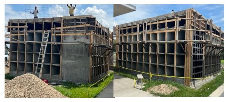
The construction phase of Mausoleum VII continues to progress. Pictured above is the forming process of Tier E.
