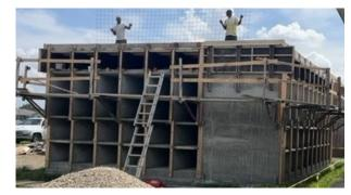
The construction phase of Mausoleum VII continues to progress. Pictured above is the forming process for the final pour of the roof.
